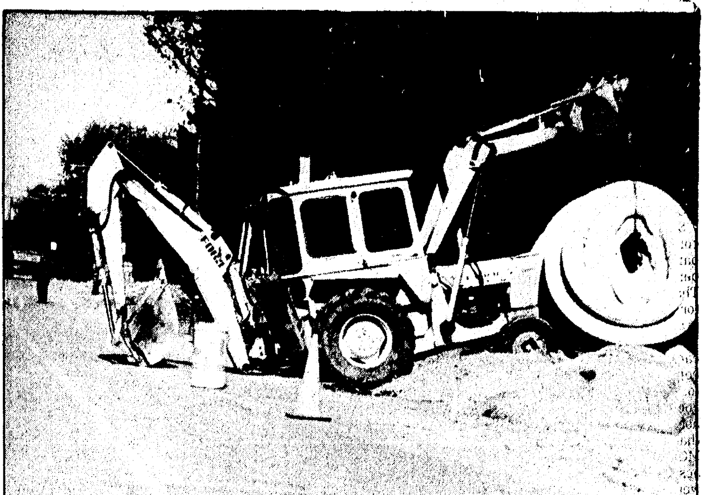
WORK IS JUST ABOUT DONE on repairs to a storm sewer drain on the north side of Sibley Rd. which backed up last fall. Village public works employees and equipment did the job.
